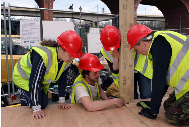
Image 3: Protohome members learning whilst building the floor (photo credit: John Hipkin)
