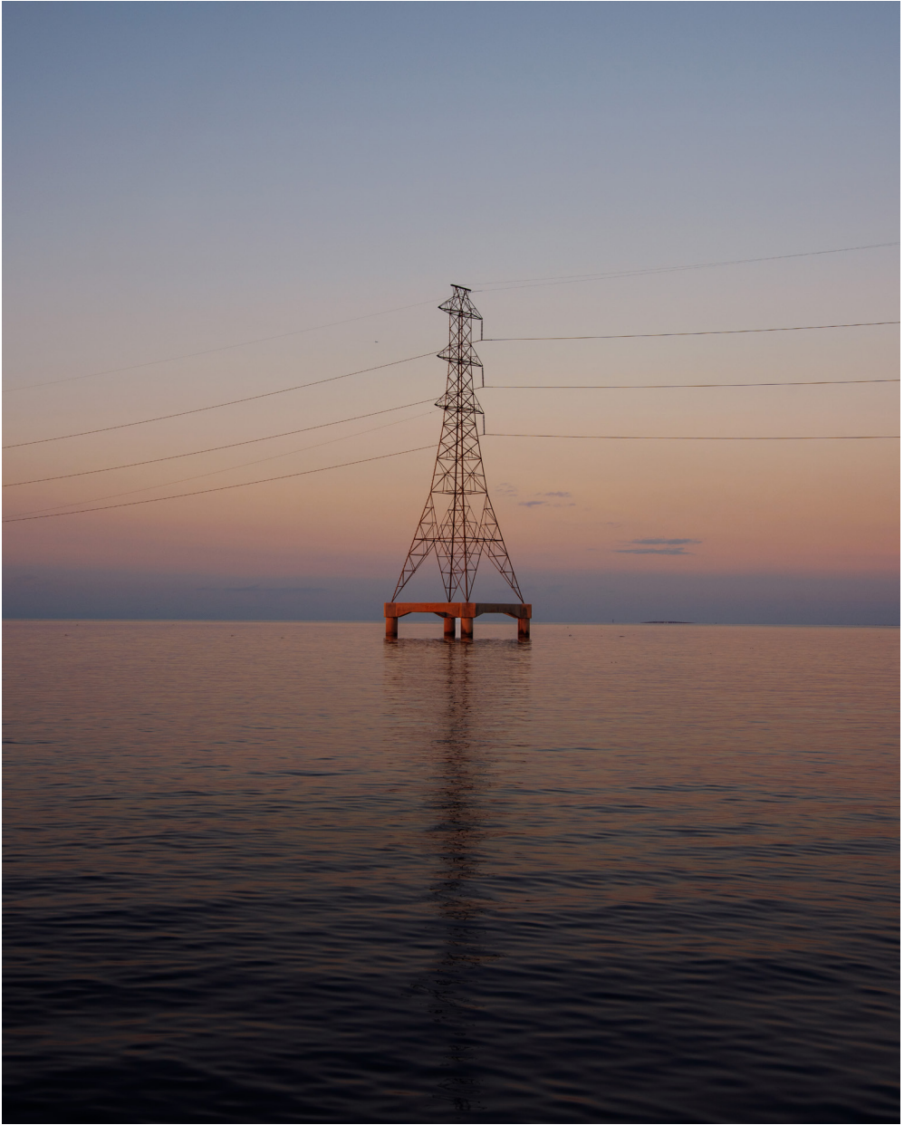
Power Lines in Kenner (2020) Copyright: Virginia Hanusik
