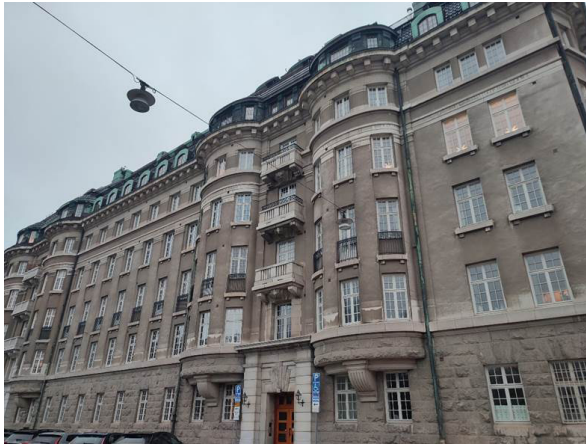
Figure #13: Bondeska Huset at Engelbrektsgatan.
