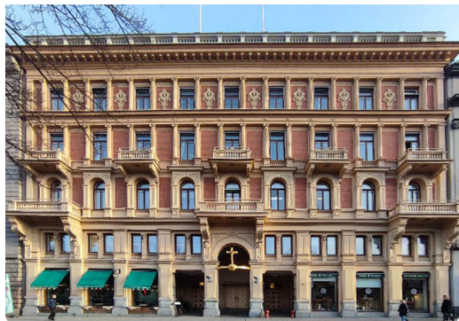
Figure #11: Catholic church for the Parish of St Eugenia today;
